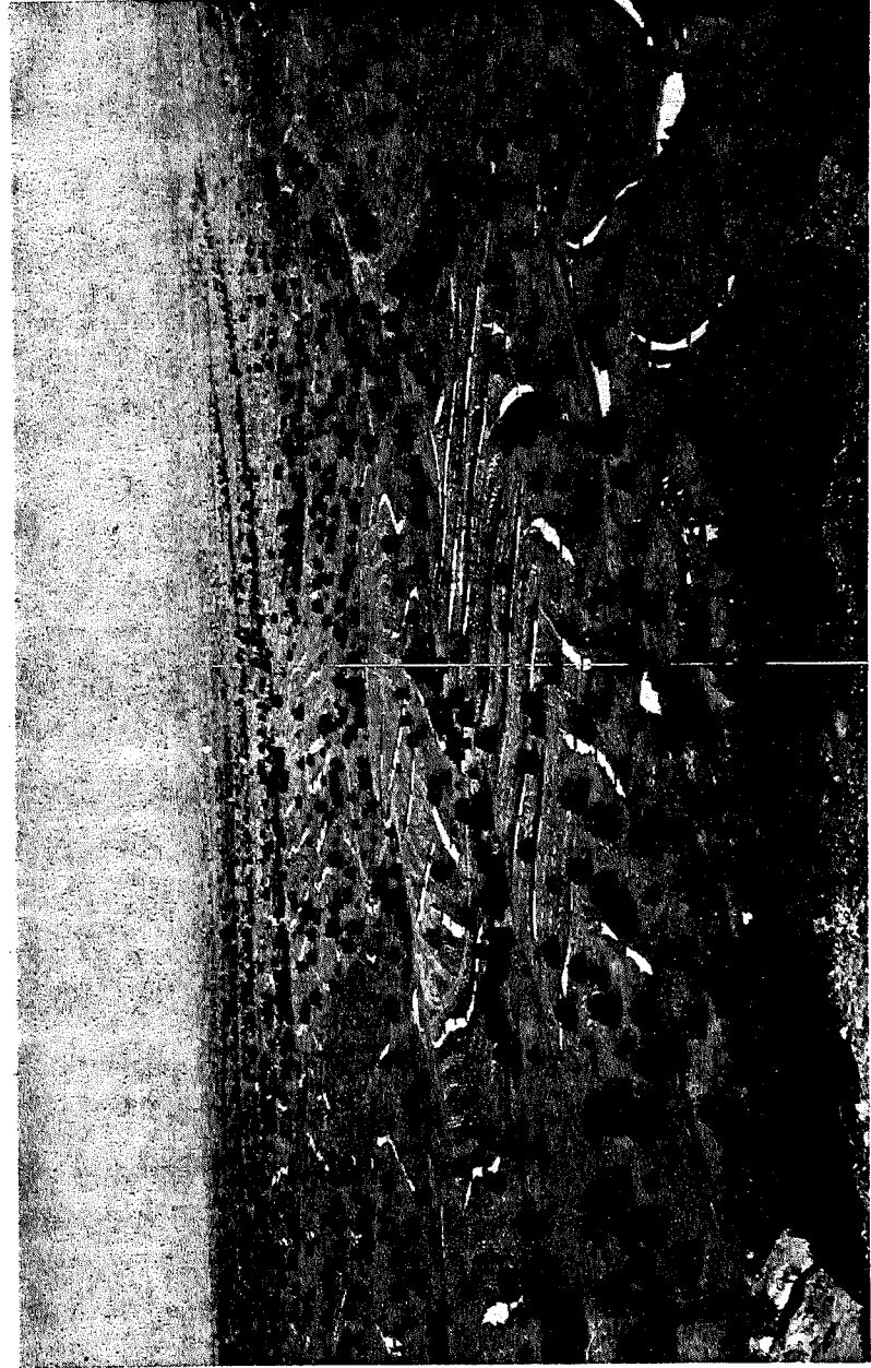
Water filled trenches on the mesa slopes above Bernalillo present an interesting pattern. Without these trenches water runs into the arroyos, carrying top soil and creating floods that do so much damage in the valley and town.
