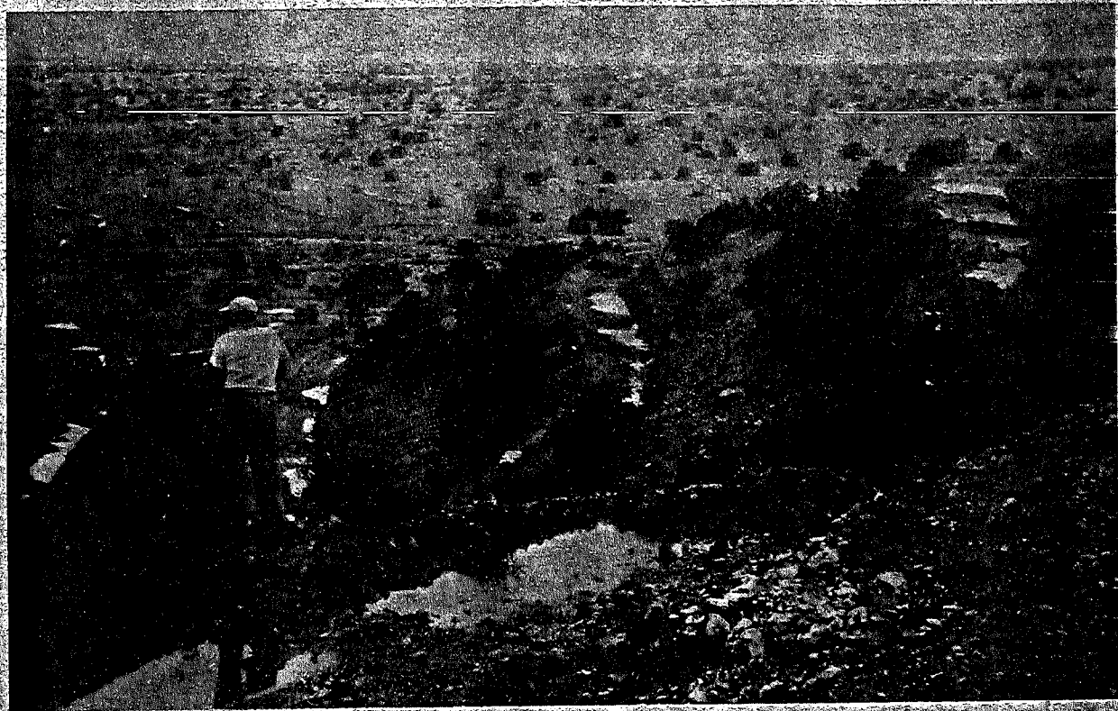
Water filled trenches on the slopes of the Bernalillo Watershed Protection Project above Bernalillo, New Mexico, from summer storms in 1955, when work was under construction. The trenches caught surface run-off, preventing floods in the community below.
