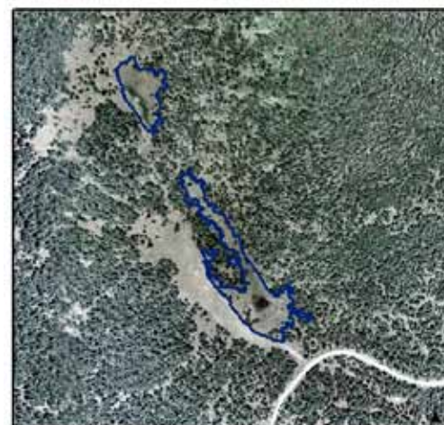
Figure G-171. Aerial photo of a representative polygon of map unit 19A.
