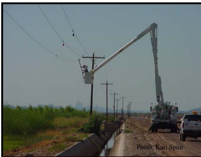
Figure 4-3 Flapper Installation
