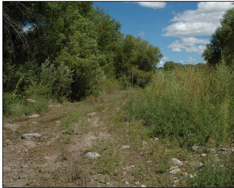
Figure 9. One of many places within the canyon where the road has been graded through the active river channel.
