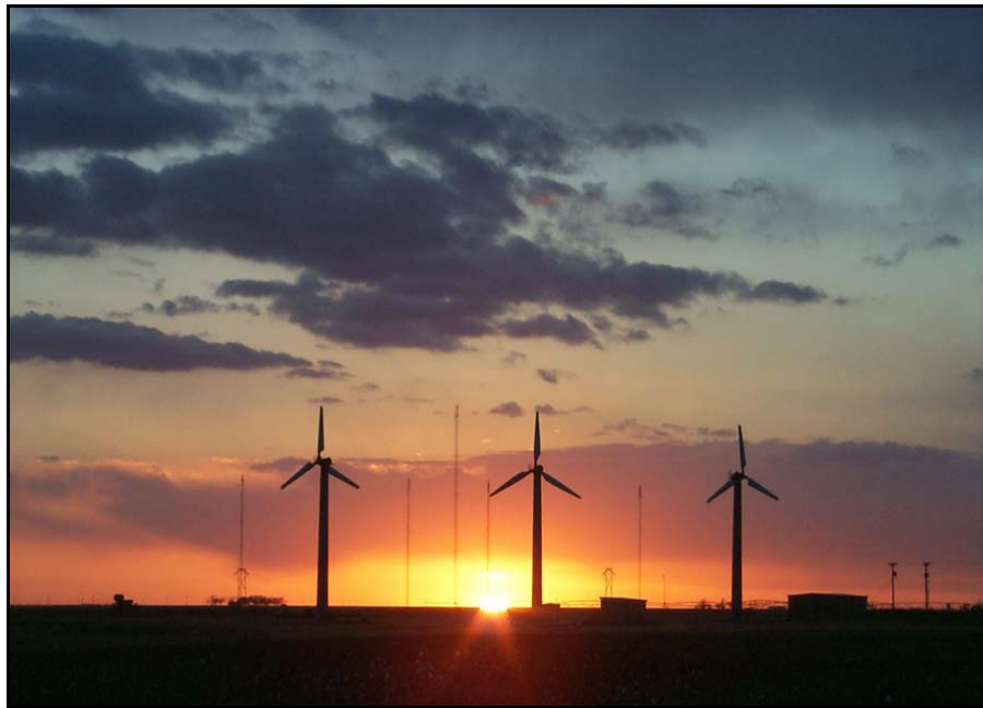
Wind Turbines in New Mexico
