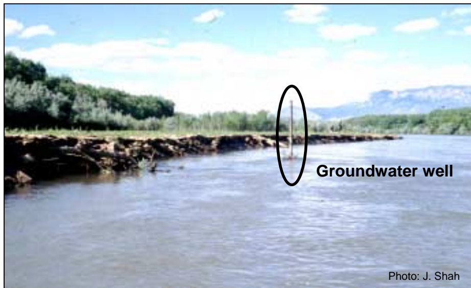
Figure 9. A groundwater well at the end of Line B was orphaned in the river by bank erosion in the first flood of 1998 (photo taken May 22).
